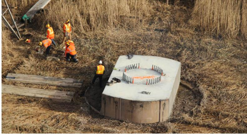
Figure 3: Value Engineered Concrete Pile Cap
