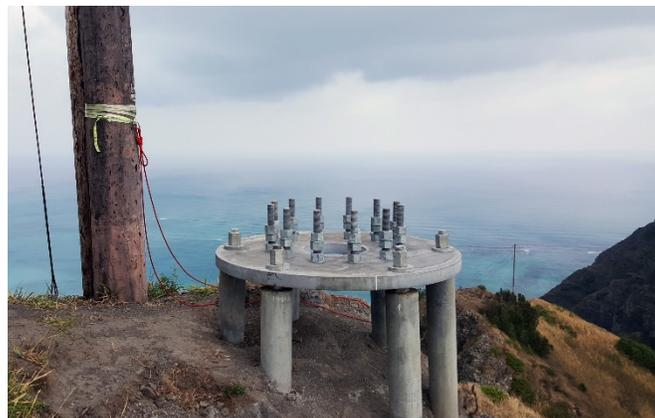
Figure 8: Installed Steel Pile Cap
