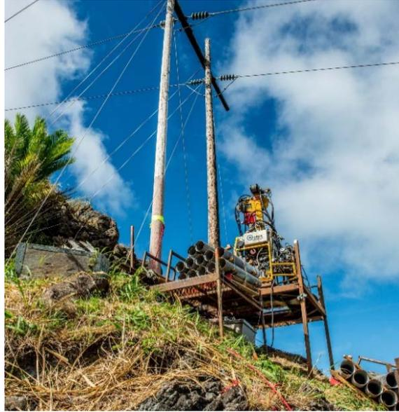
Figure 7: Steep Slope Configuration
