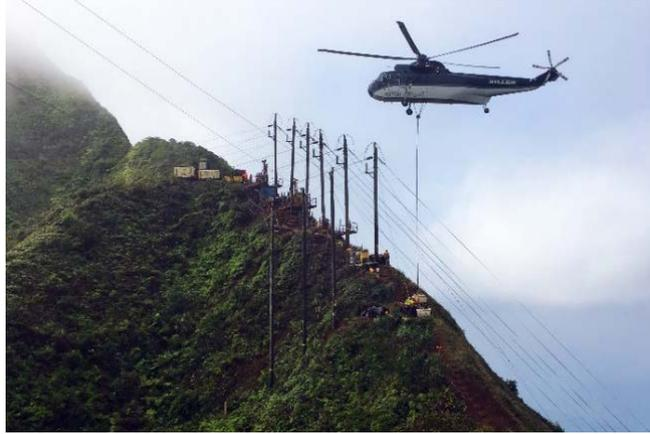
Figure 5: Helicopter Transporting Material to Foundation Sites
