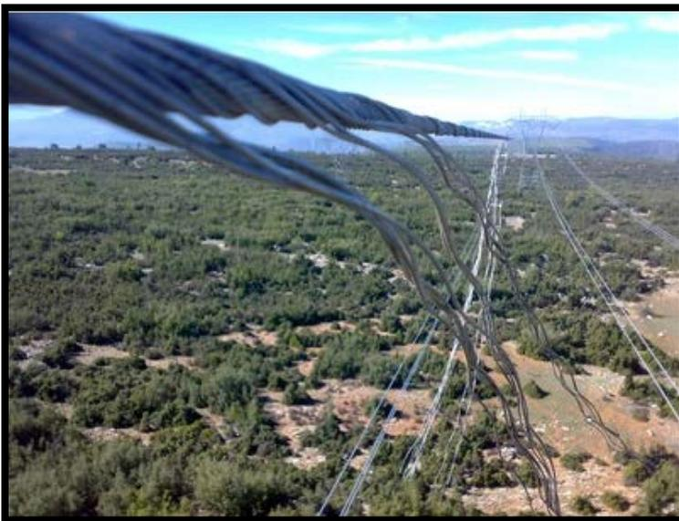
Figure 10. Transmission line shield wire showing evident damage in need of replacement
