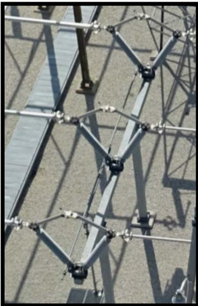
Figure 2. Center Break Switch Inspection
