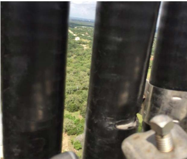
*Figure 13. Microwave tower cabling damage*
