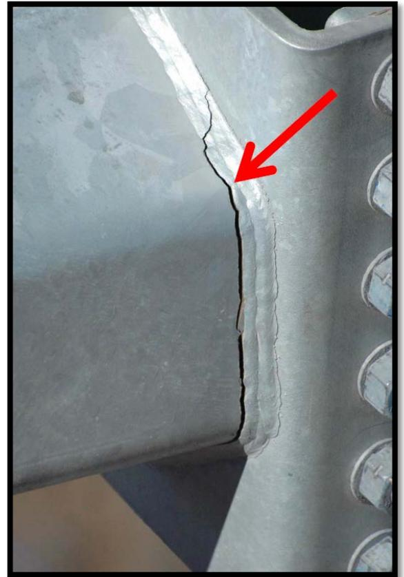
*Figure 11. Cracked joint at arm of transmission line structure*
