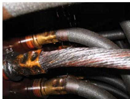
**Figure 5** - Overheating of Connection #7
